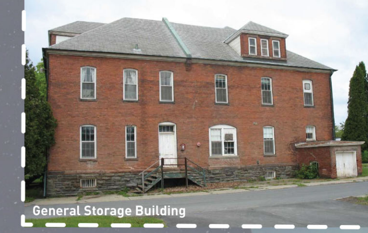
General Storage Building
