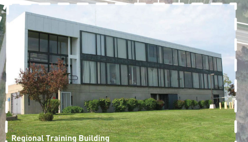
Regional Training Building
