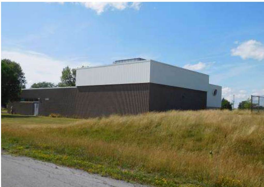
BUILDING #744 – GYMNASIUM/RECREATION CENTER
