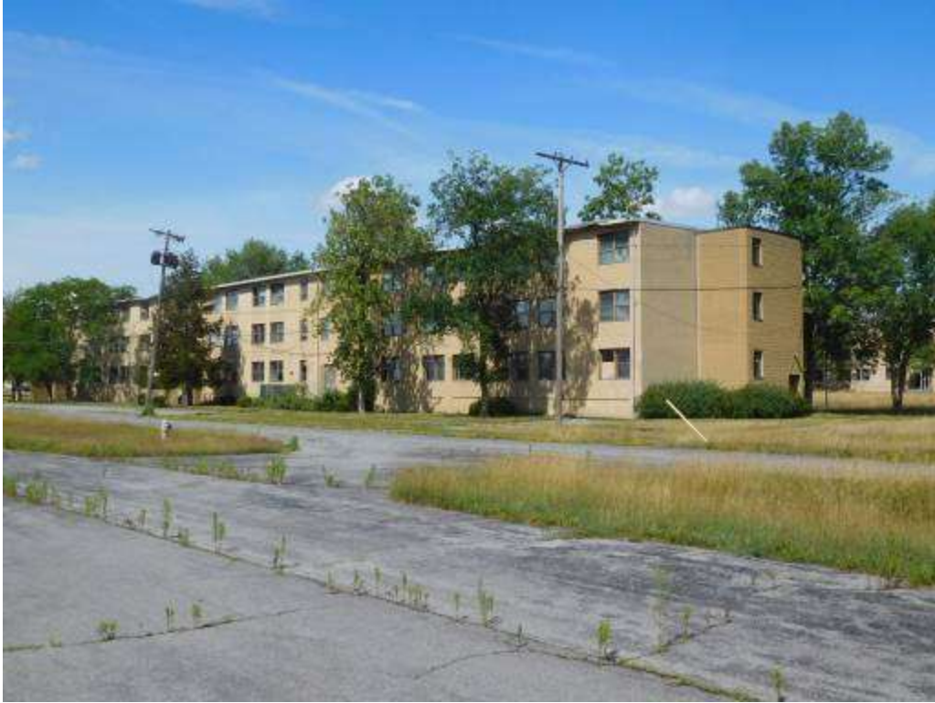
BUILDING #709 – OLD ARMY BARRACKS BUILDING
