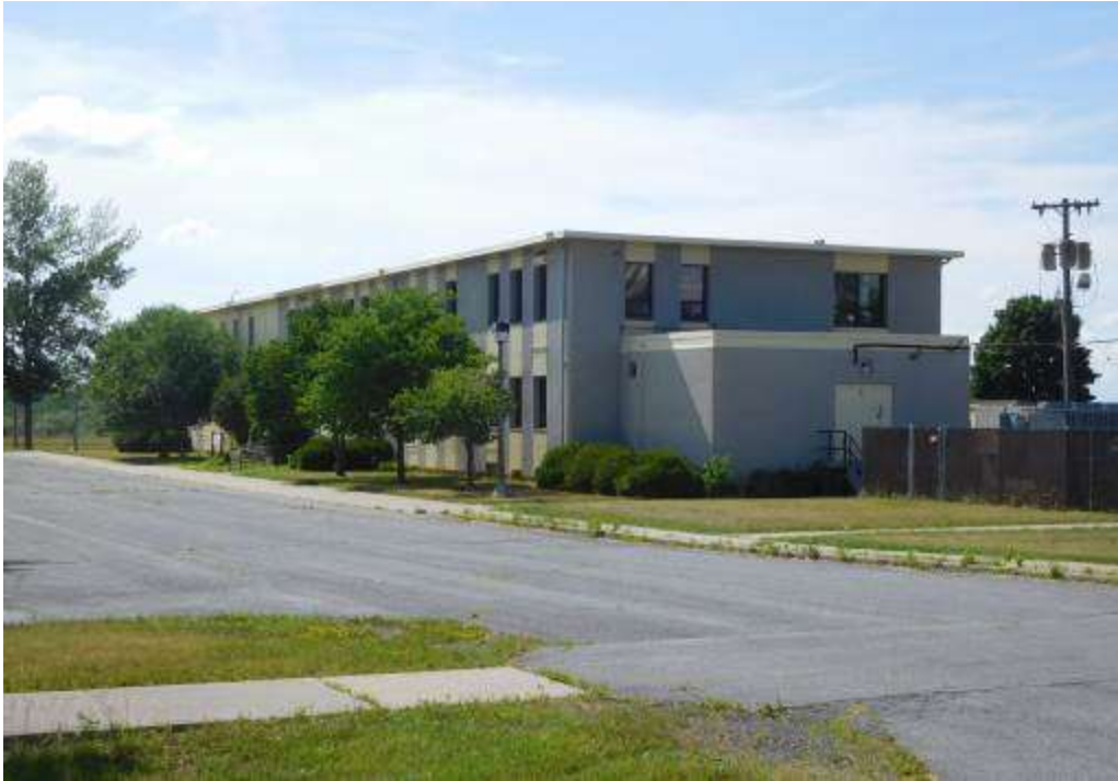
BUILDING #701 - LANGSTEN HUGHES HALL SCHOOL BUILDING
